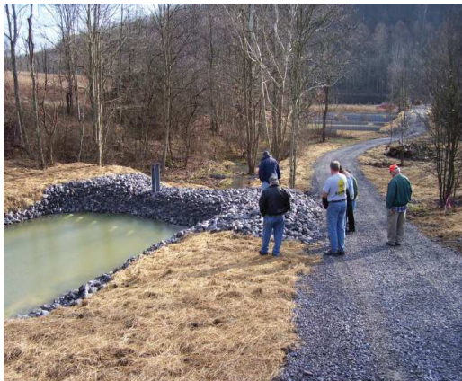
Figure 2. Water gains alkalinity as it flows through a leach bed at Site 3
